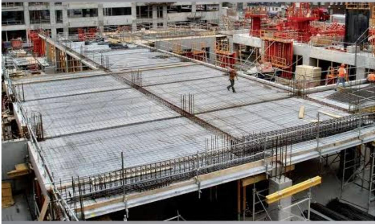
Figure: 4. Hybrid concrete construction
