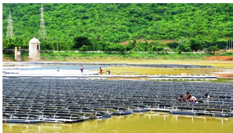
Fig: Floating solar power plant started location is Mudasarlova, Arilova, VSP District
