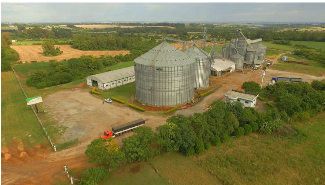
Figure 7 Cotribá facility at Santa Margarida.
