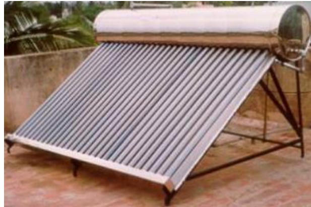
Fig. 2: The evacuated tube collector type device.
