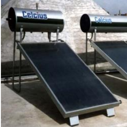
Fig. 1: The flat plate collector type device.
