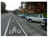
**5. Right angle parking:** In right angle parking or 90° parking, the vehicles are parked perpendicular to the direction of the road. Although it consumes maximum width kerb length required is very little. In this type of parking, the vehicles need complex manoeuvring and this may cause severe accidents. This arrangement causes obstruction to the road traffic particularly if the road width is less. However, it can accommodate maximum number of vehicles for a given kerb length.
