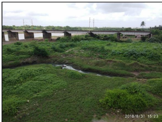
Figure 4 View from the Auranga river bridge
