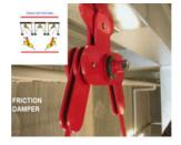
Using rotational friction dampers in retrofitting
