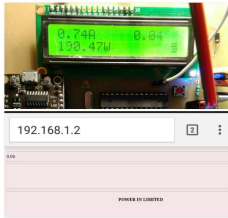
Figure 4. Meter status at normal condition
